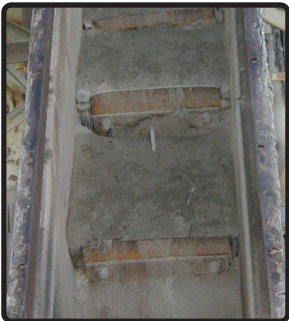
AR Steel Liner
