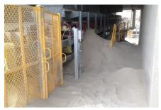
An operation's load zone was not properly supported which allowed the belt to porpoise between the impact idlers. Significant spillage, dust and maintenance resulted from this issue. The Load Zone was running 3000TPH with two Cone Crushers at 1,100hp each, crushing 14" minus material to 34" minus. A three-man crew spent six hours twice a week cleaning up the spillage.
