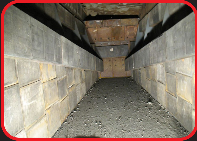
Completion of Installation
