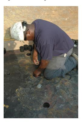
After you have finished welding the studs through each mounting hole, you will need to drop a flat washer over each stud, followed by a nut, and then securely tighten using a pneumatic impact wrench.
