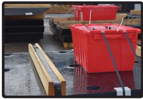
Liners are pre-palletized and stacked for easy installation. The necessary hardware is secured in sealed containers.
