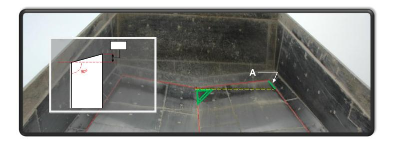
You will need to measure the end of the line to the corner of the floor and the cant, to get the dimension for "A".
