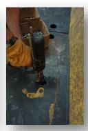
After you have finish welding the studs through each mounting hole you will need to drop a washer over each stud followed by a nut and then securely tightened using a pneumatic drill.
