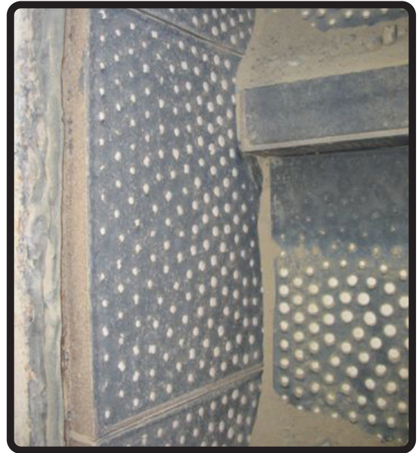
Rubber-Ceramic Liner
