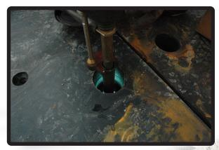
A stud welder gun provides a quick and strong method for applying the threaded studs to the steel floor through the counterbored holes.
