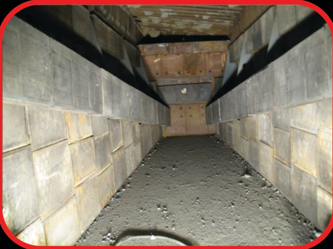
Completion of Installation
