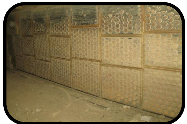
Discharge wall in a 60" feeder
